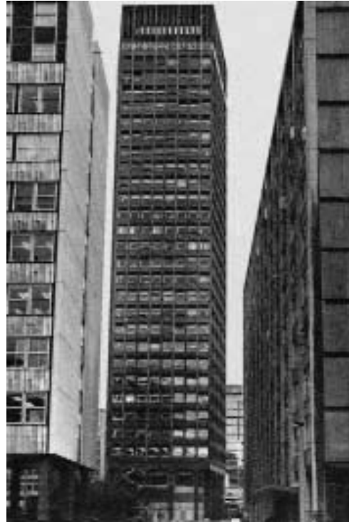
Figure 4.11 Office development, City of London
